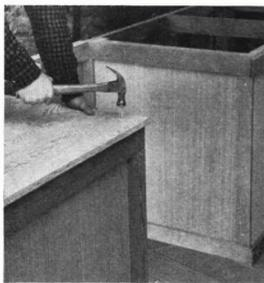
Make counter top of 3/4-inch exterior grade plywood, leaving about an inch overhang. Fasten it with aluminum drivingscrews, or 2-inch brass screws
