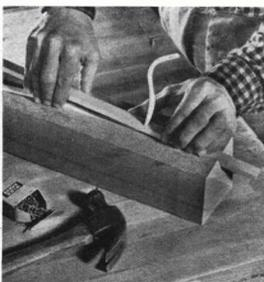
Cover wire in groove with strip of wood held with brads. Wire should be installed before the post is set. Have electrician make the connection
