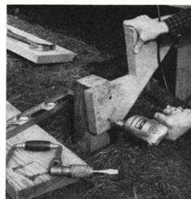
Terrace should be about 8 inches off ground. If ground slopes on approach side, make one step for each 8 inches of rise, using planks 2-by-10 or wider
