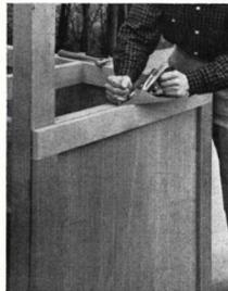
6 Finish terrace with two coats of penetrating resin sealer, available in many colors, or with deck paint. 7 Storage counter is made of thin exterior-grade plywood (over framework detailed on next page) with 1-by-3 trim nailed over it. Use plane to smooth trim and to make top level before counter top goes on
